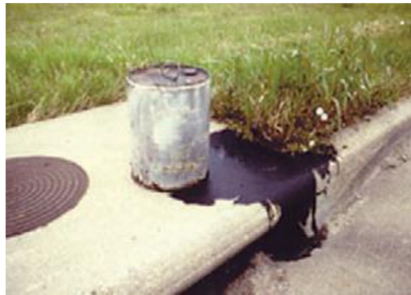
Dumping at Storm Drain Inlet
