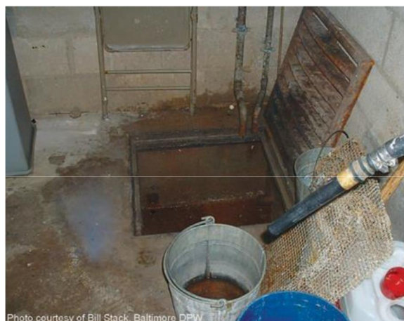
Cross-Connected Floor Drain
